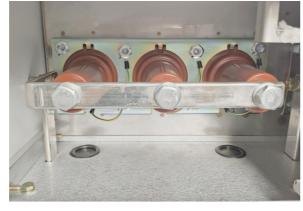
breaker switch is in the ground position. This interlocking mechanism prevents accidental access to the test access during operation. The test sleeves in the facility are grounded using a grounding rod, which needs to be removed to isolate the test sleeve from the ground connection prior to performing cable testing. Test ports can be used for cable testing and fault location without removing cables and reducing power system downtime.
